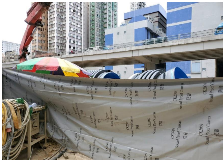
Figure A2 Noise barrier mat erected for grinder
