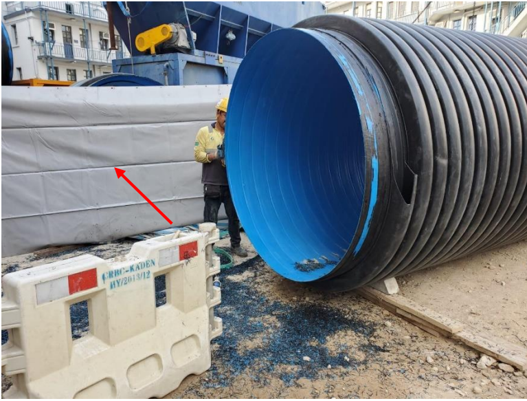
Figure A3 Noise barrier mat erected for grinder
